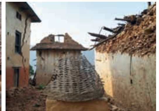
Raghuchour village, after the earthquake
