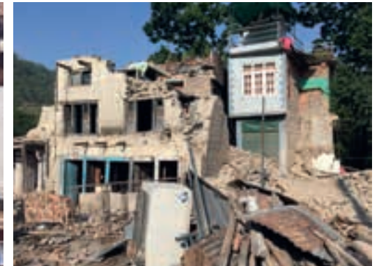
Raghuchour village, after the earthquake
